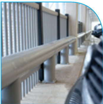
Car Park Barrier with Anti-Climb
